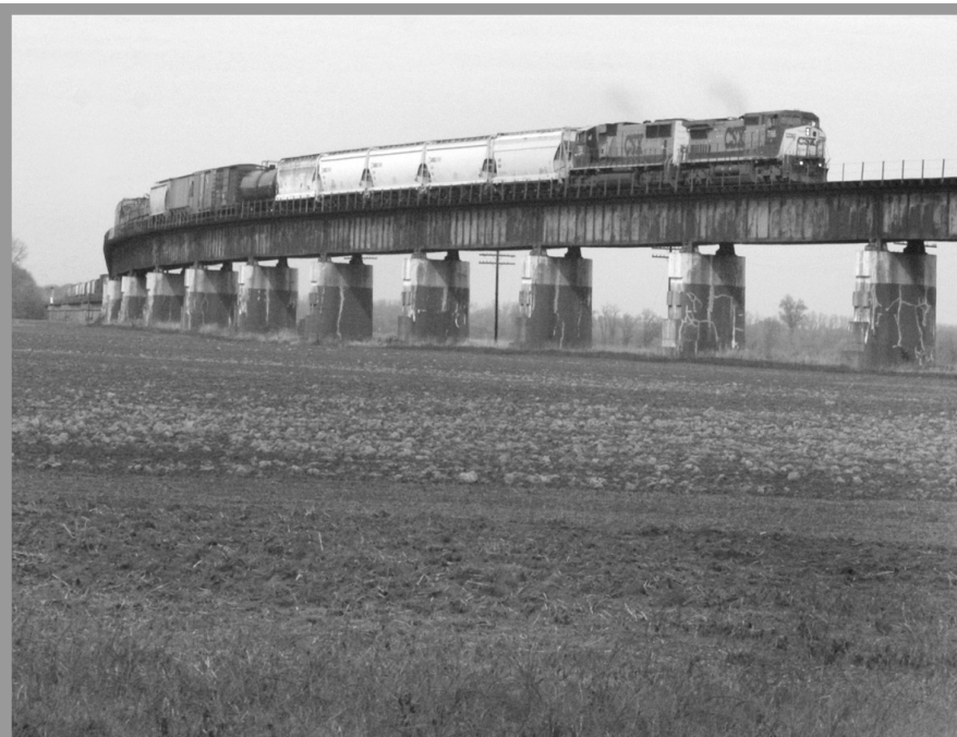
A CSX manifest winds it's way slowly over the north approach to the Henderson Bridge over the Ohio River. This bridge connects Evansville, IN with Henderson, KY. Jim Pearson made this shot in the spring of 2003, as a part of his continuing study of CSX's Henderson Sub. photo by jim
